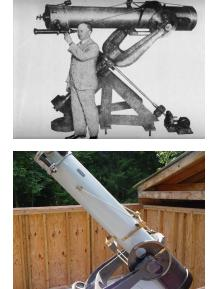
He designed and largely constructed a 12-inch reflecting telescope in 1929. This equatorially mounted instrument is housed in a sliding roof observatory on the roof of his factory. Before the Cold War, a copy of the Patton telescope was made from his drawings by the Russians and was mounted in a small observatory in Neish Novgorod.
